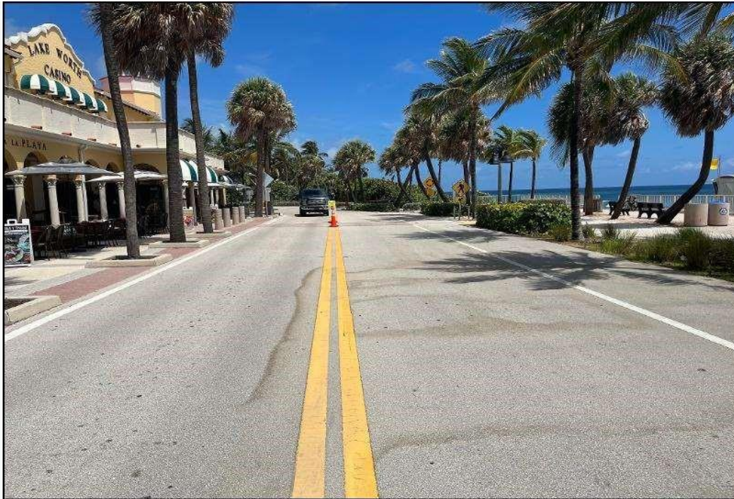
Access Road facing north
